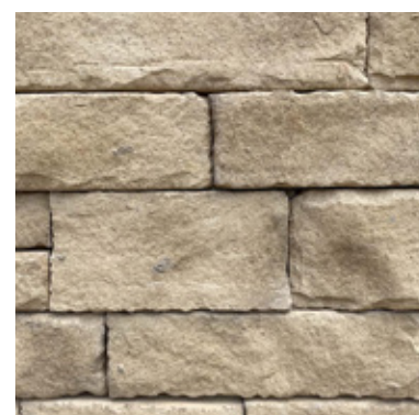
DRY STACK GRAND CANYON
